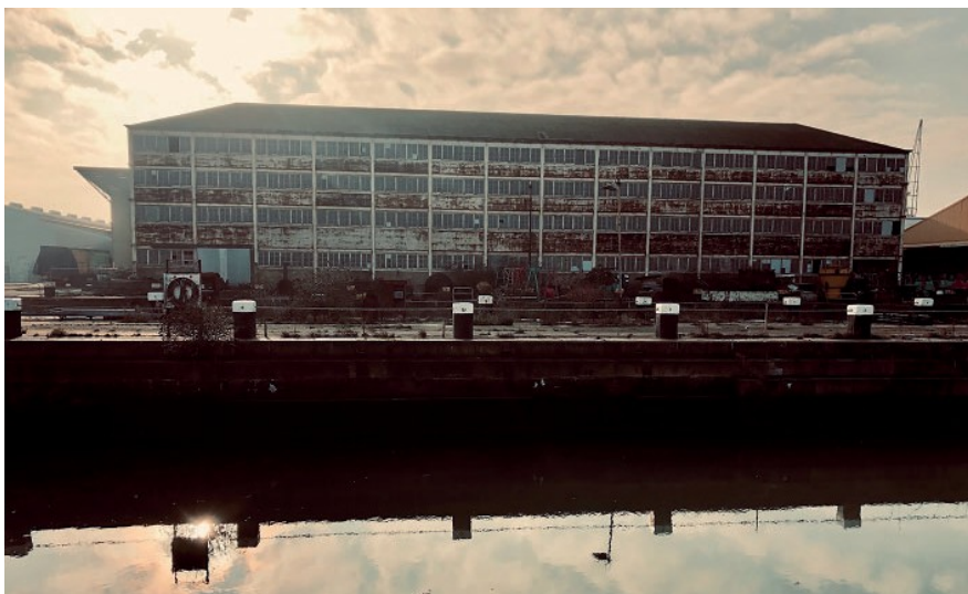
Boat Store at Sheerness Port – Heritage at Risk Grade I listed building
