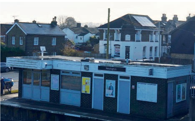
The modern replacement station and adjacent Victorian
