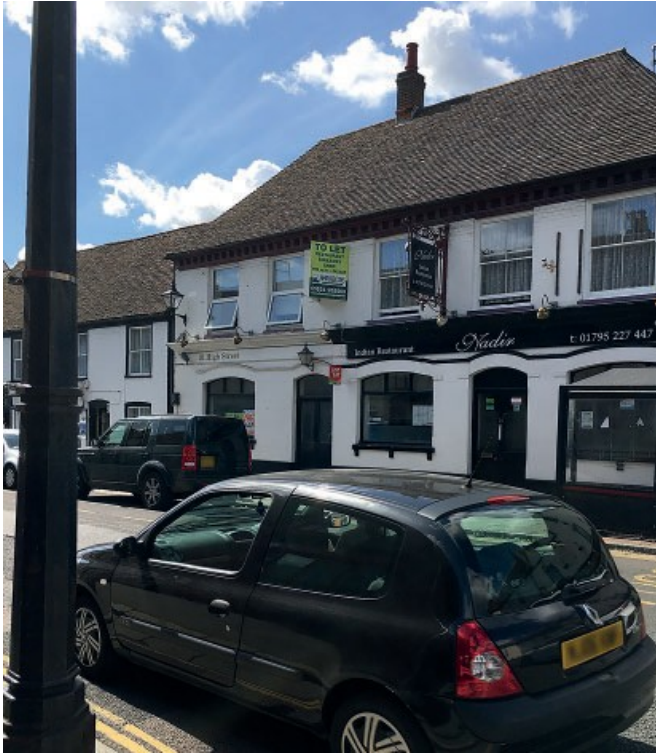
89-91 High Street, Milton Regis (a grade II listed building).
